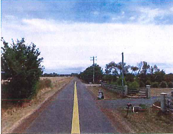
Figure 24 – Looking north along Bishopsbourne Road from Balance Lot
