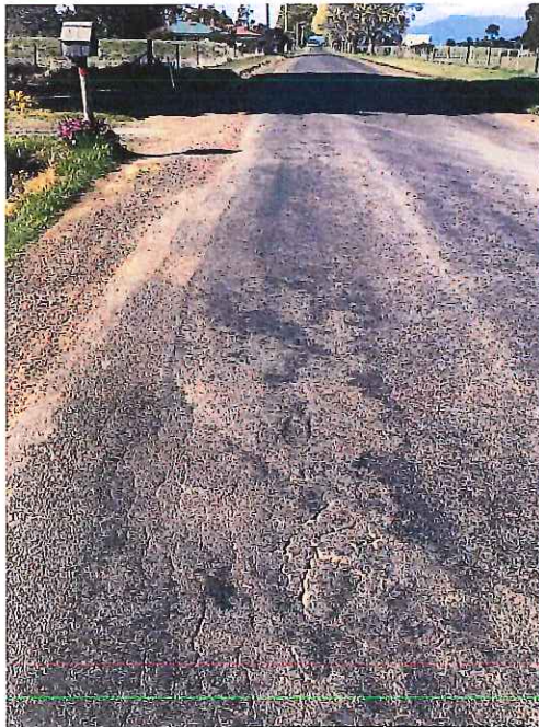
Figure 13 – Bishopsbourne Road seal condition north side of Coach Lane junction
