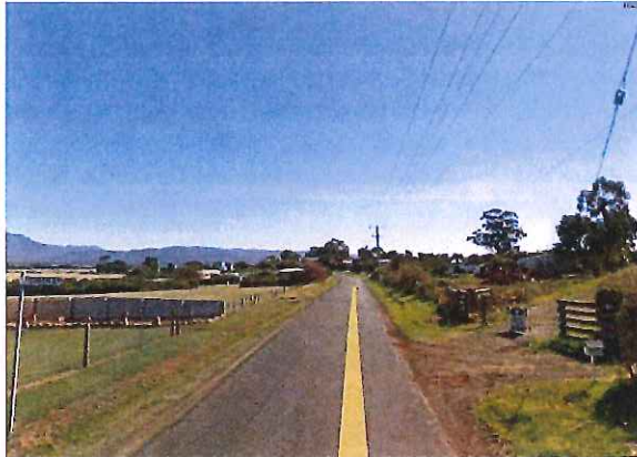
Figure 19 – Looking west along Bishopsbourne Road from Coach Lane (West end)
