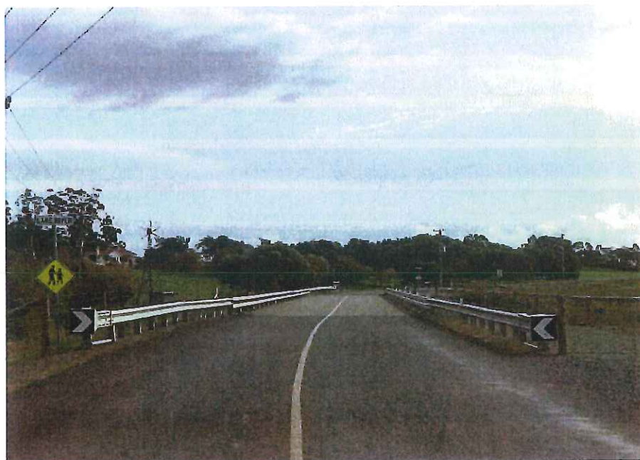
Photo 4 – View of the new 2-lane Lake River bridge constructed 900m to the west of Pisa Bridge
