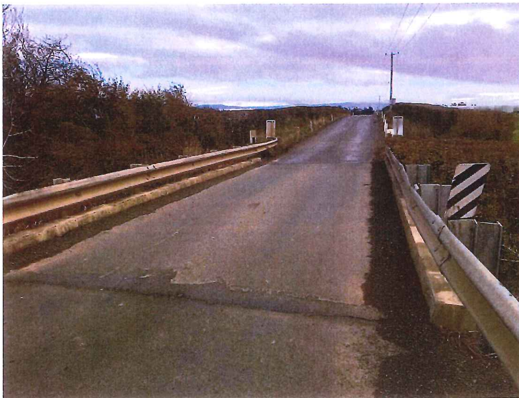
Photo 1 – View of Existing Bridge at Deck Level
