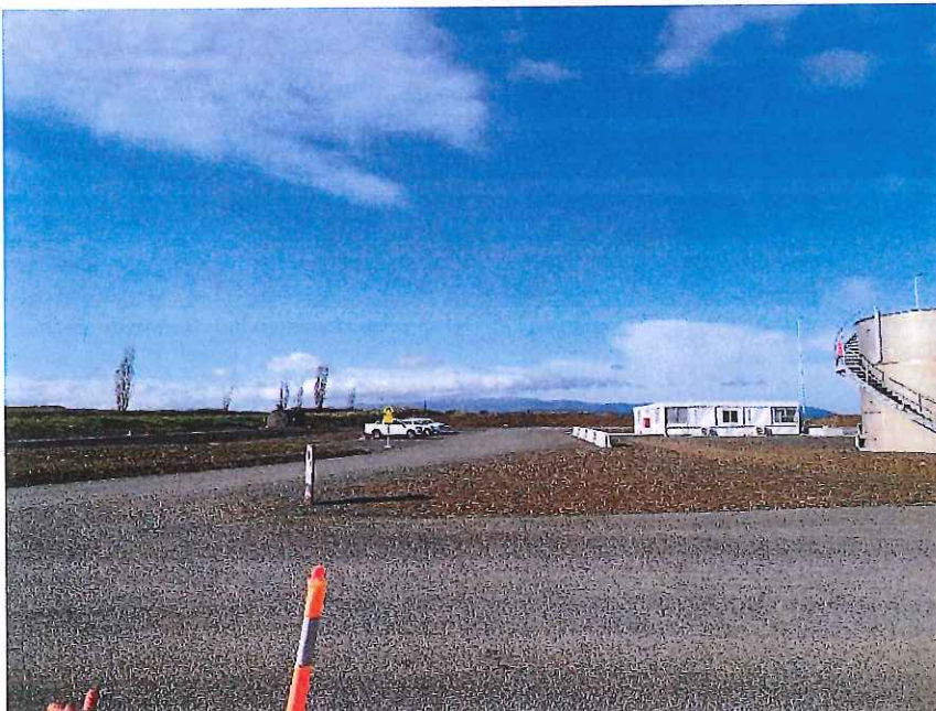
Figure 2 – site entrance looking north
