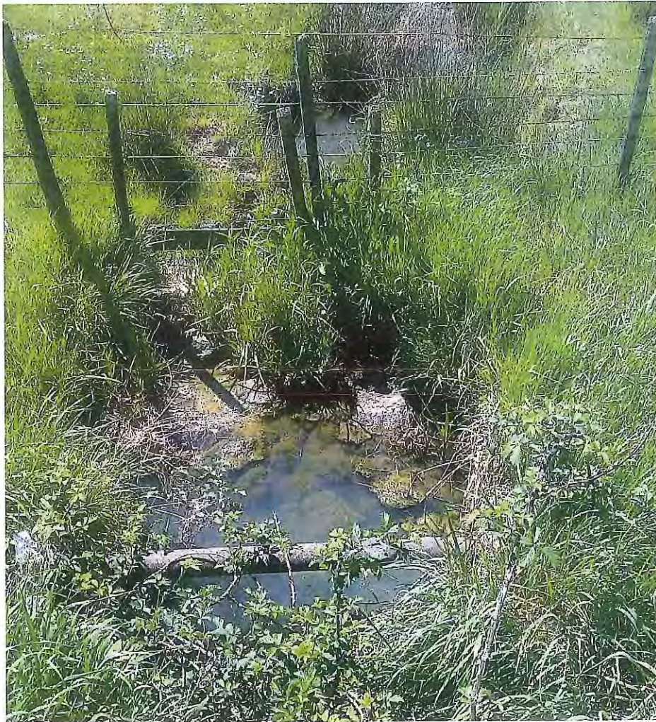
Plate 3: Drain at culvert outlet
