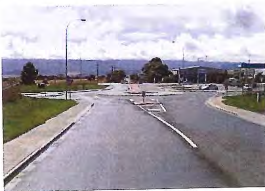
Figure 4: Translink Avenue facing north-east (Source: Google Earth January 2010)
