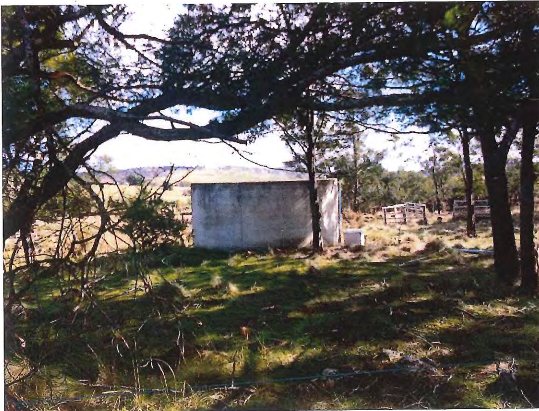
Figure 9: water supply existing dwelling lot 3
