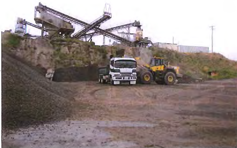
Photograph 4: Primary crushing and screening plant in operation
