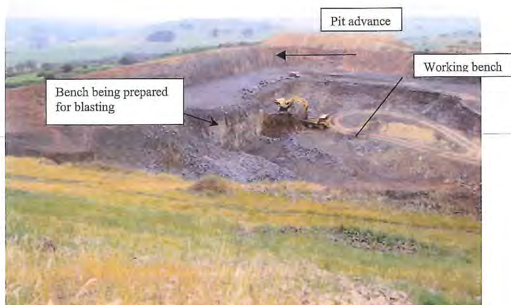
Photograph 1: Typical quarry bench operation. Quarry advances to the left
