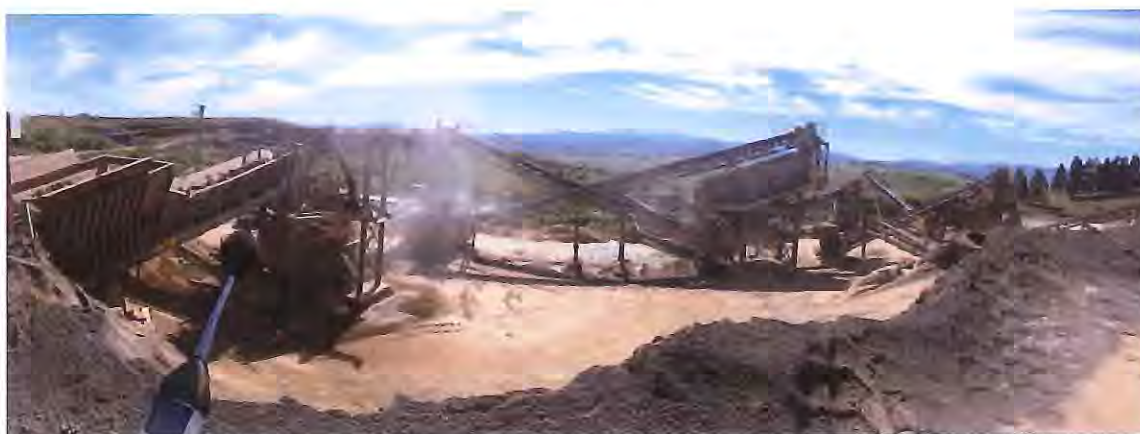
Figure 2: Crushing Plant – Looking East from Crusher Inlet
