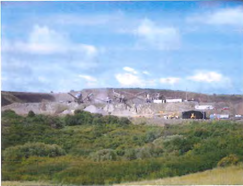
Photograph 3: View of crushing and screening plant in operation
