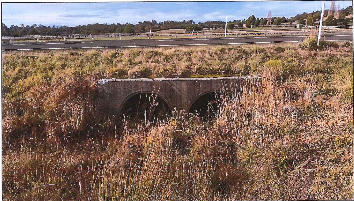
Image 4 – Existing twin DN1050 concrete culvert under old highway
