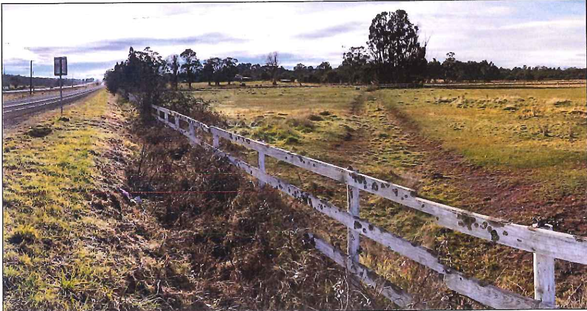
Image 2 – Existing drainage channels extending north east from existing culvert
