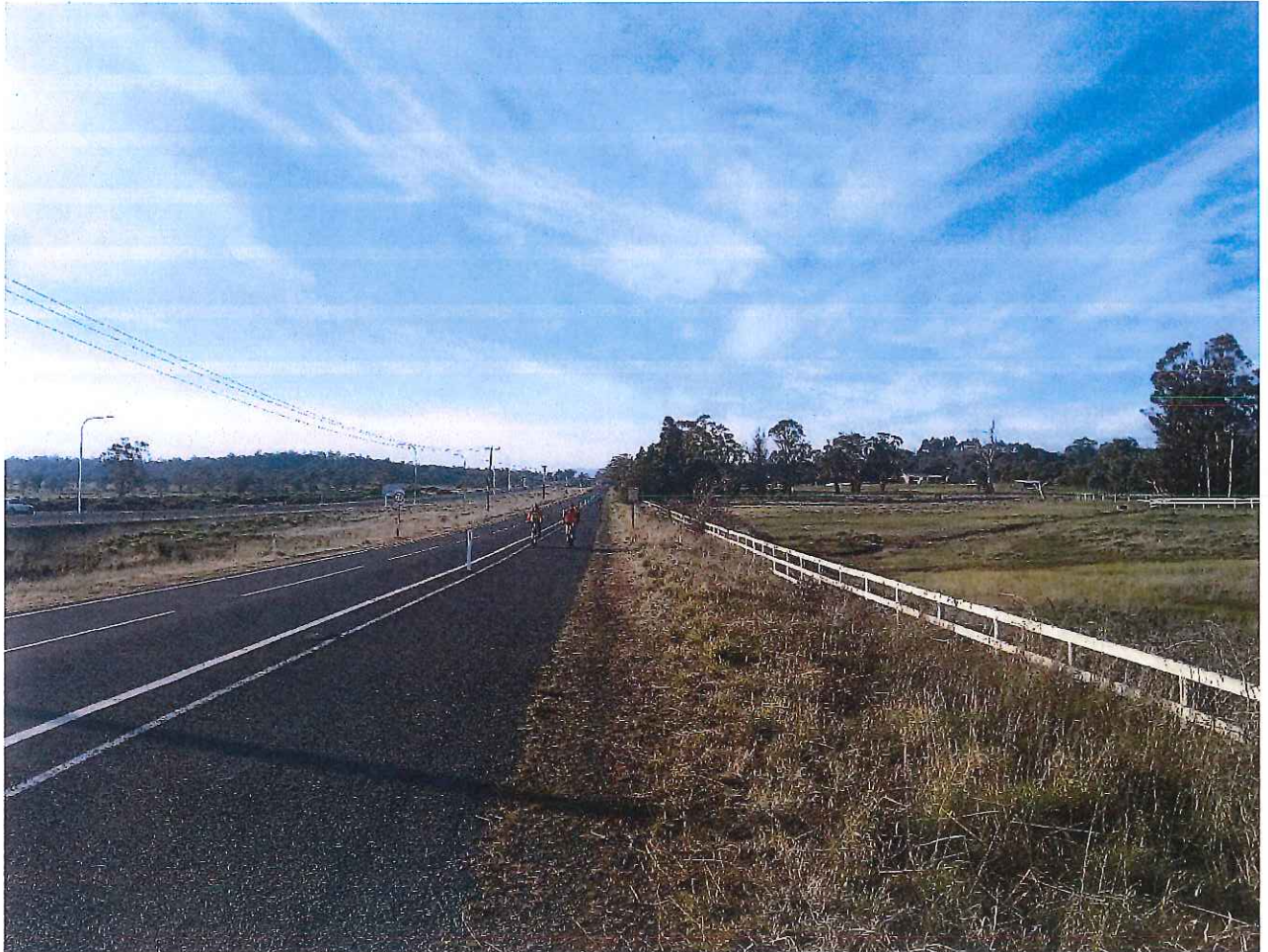
Image 3 – Looking north along Haggerston Road. Available sight distance is in excess of 750m from the proposed intersection on the righthand side.
