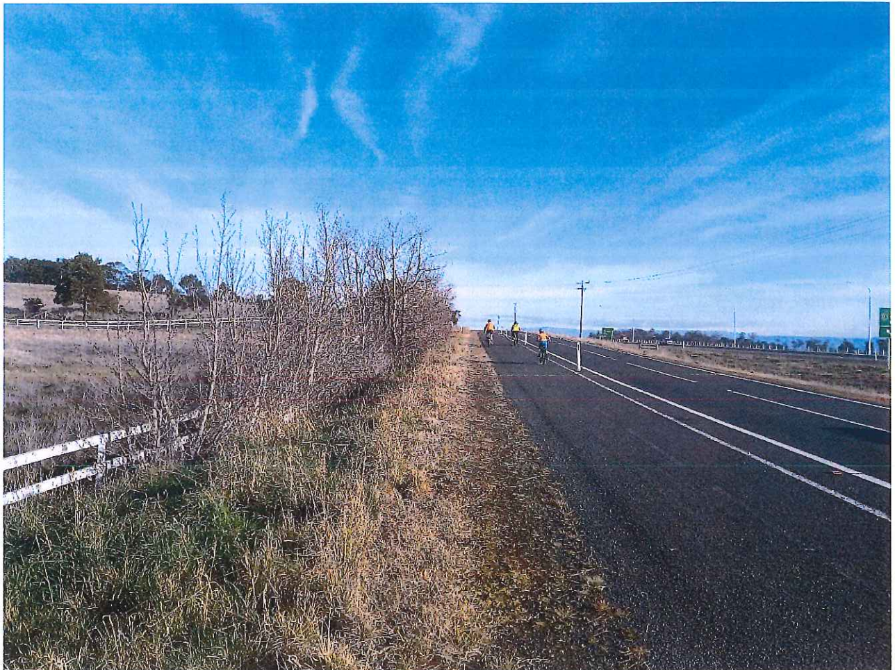
Image 4 – Looking south along Haggerston Road. Available sight distance is in excess of 280m from the proposed intersection to the crest adjacent to the Gibbet Hill Rise intersection.
