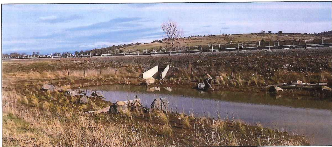
Image 3 – Existing wetland and culvert under new highway
