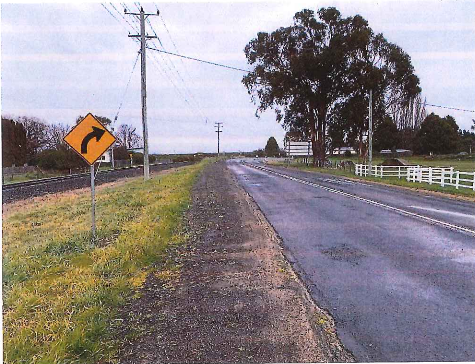
IMAGE 1 - Southbound approximately 100m from 158 Illawarra Road
