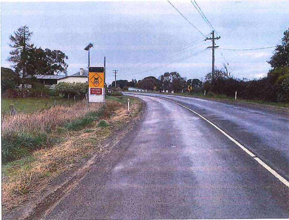
IMAGE 3 -Eastbound approximately 45m from 158 Illawarra Road
