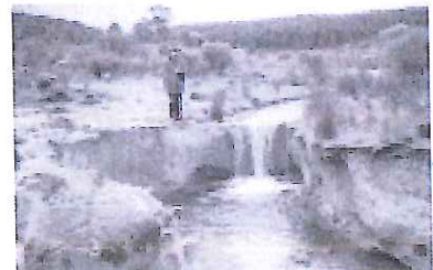
Headcut eroding stream bed
