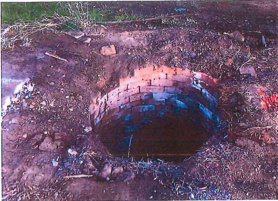
Photo 3 – View of well from NE
