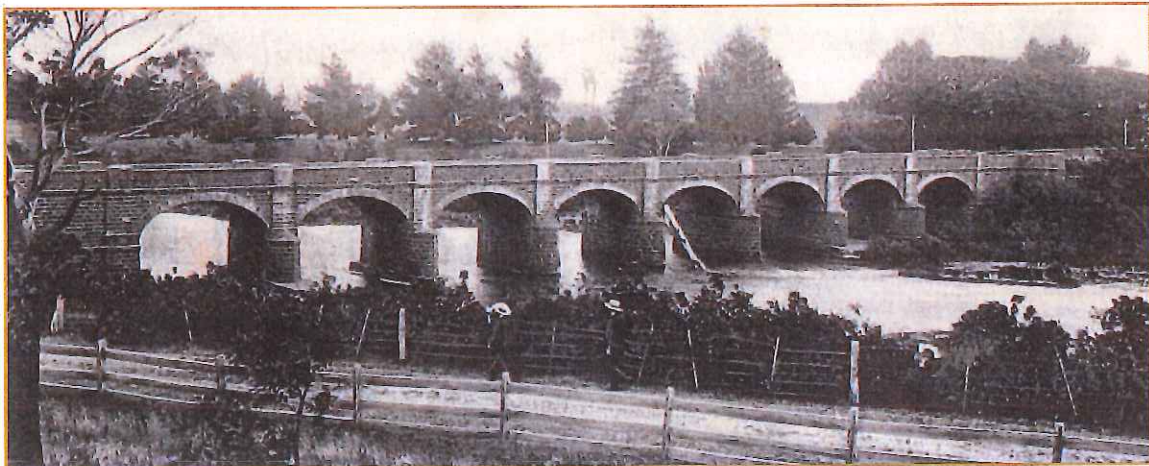
Figure 22: Early photo of Perth Bridge. Source: Libraries Tasmania 2020.
