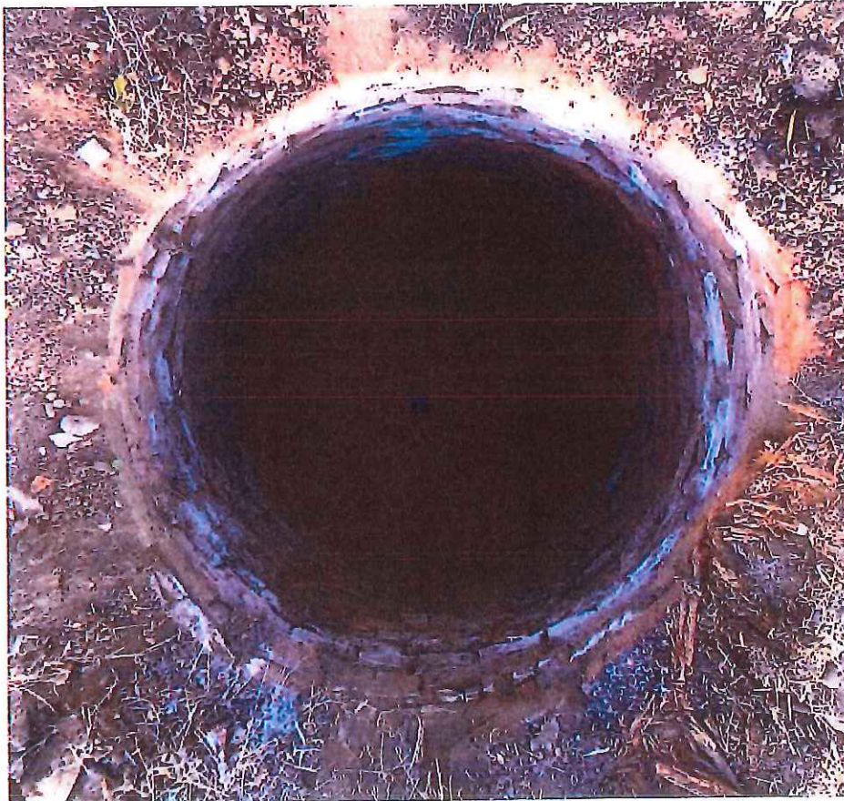
Photo 4 – View down well
