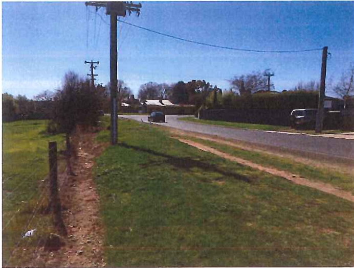
Fig 4.1c – Sight Distance from Lot 9 access (worst case) to North, considering potential sight distance to nearby intersection with Frederick Street
