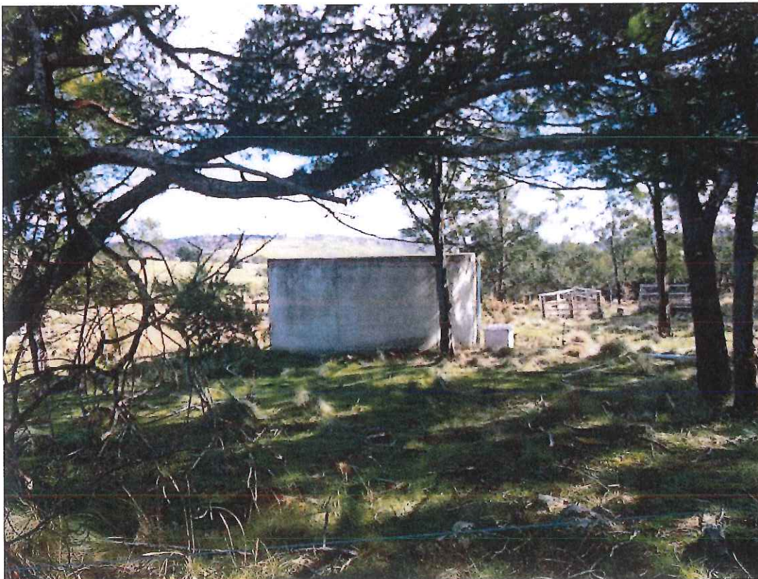
Figure 10: water supply existing dwelling lot 1
