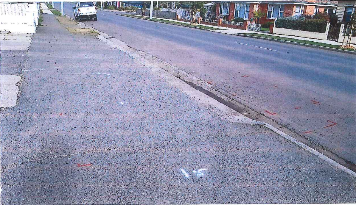
Figure 9: Red outline on roadway is possible underground petroleum tank
