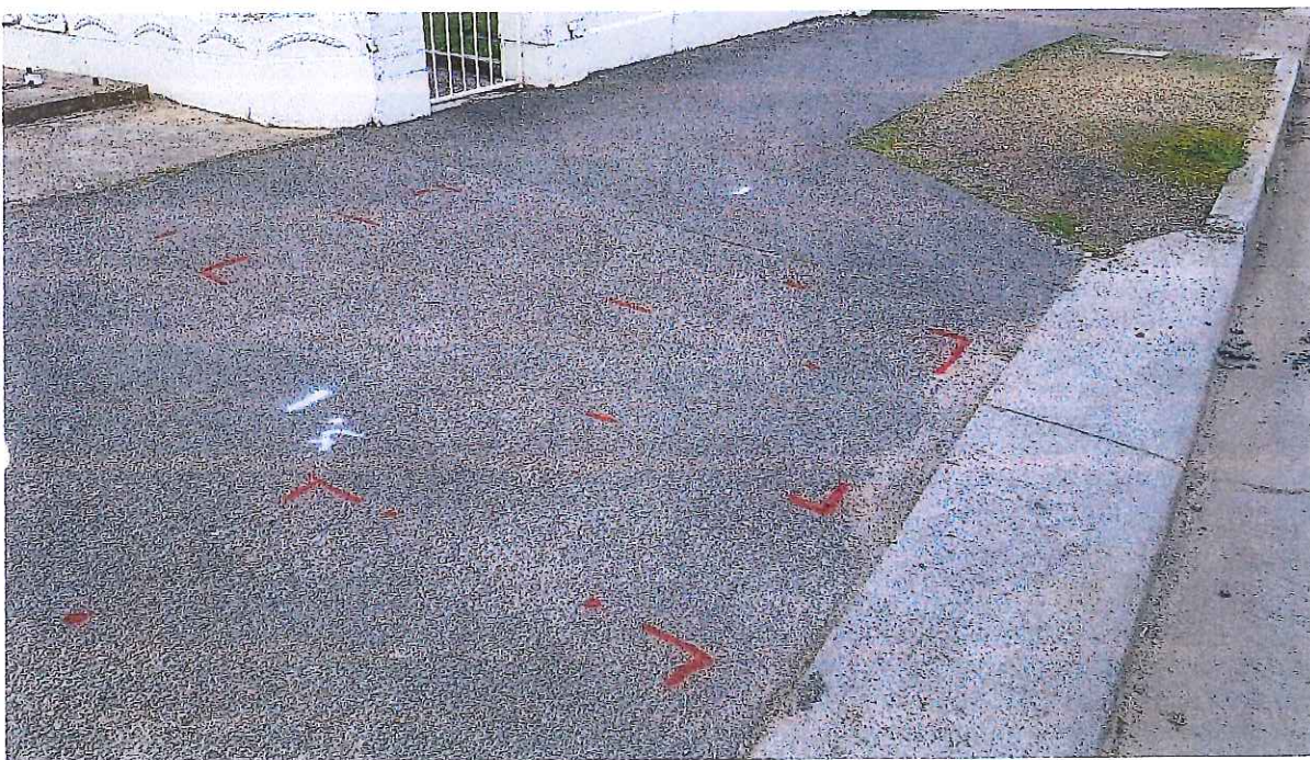
Figure 10: Red outline on footpath are indicating the presence of two possible underground petroleum tanks
