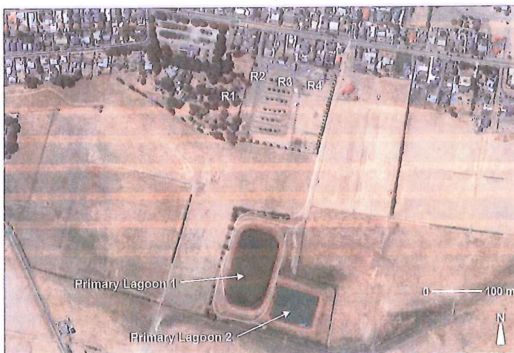
Figure 7-1: Aerial view of Evandale STP with a marked-up model emission source overlay and discrete receptor locations.
