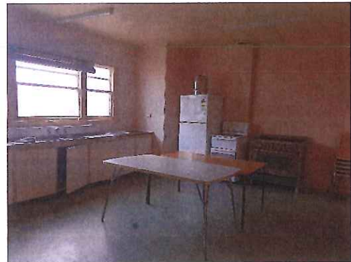
Image 7: Downstairs Kitchen Facilities 1 of 2
