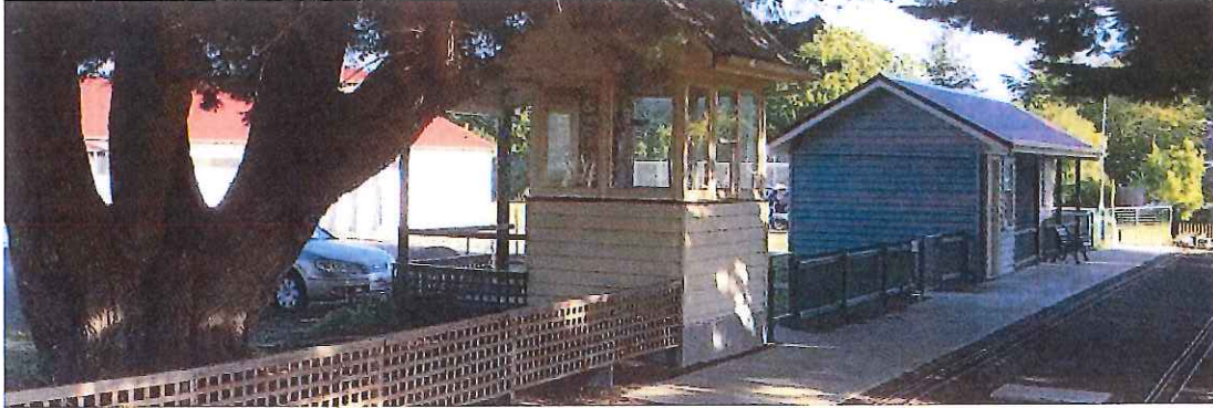
Figure 26 – Existing miniature railway station and control building.
