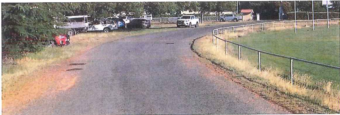
Figure 12 – Internal roadway between Barclay Street and the school car park area.
