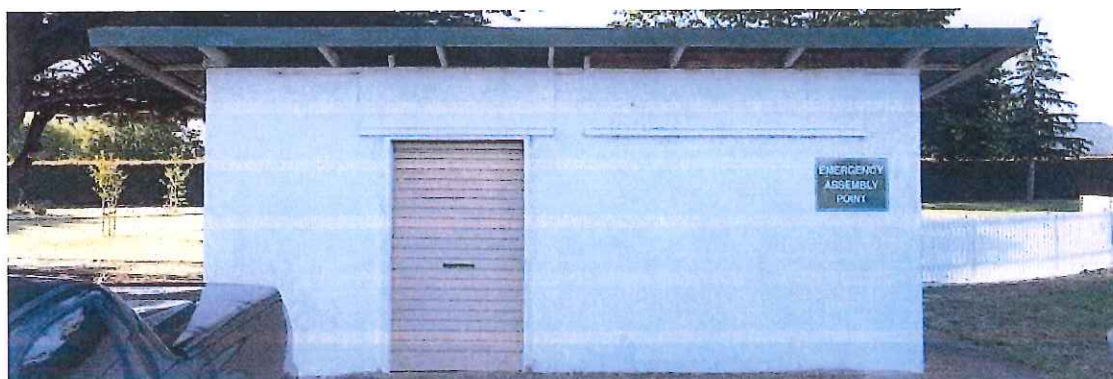
Figure 23 – Existing old change room.
