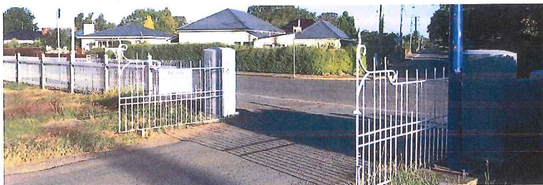
Figure 9 - Barclay Street main entry.
