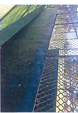
Example of rubber material for netting Image courtesy of InsideEDGE Sport and Leisure Planning
