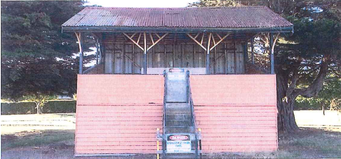
Figure 24 – Existing old pavilion.
