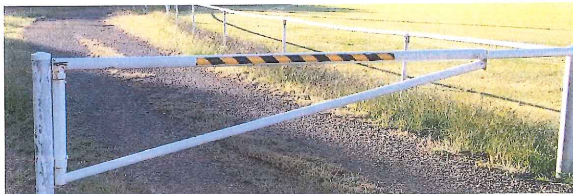
Figure 13 – Existing gate restricting access around the gravel loop road.
