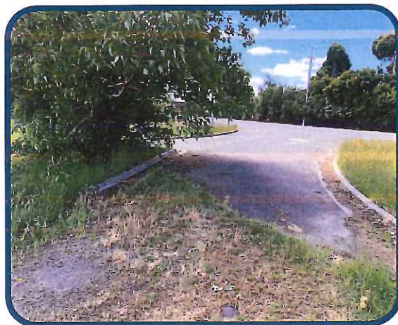
Figure 16 - Slip road in the north, onto Evandale Road.
