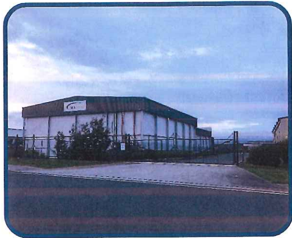
Figure 6 – Warehouse development within Translink area.
