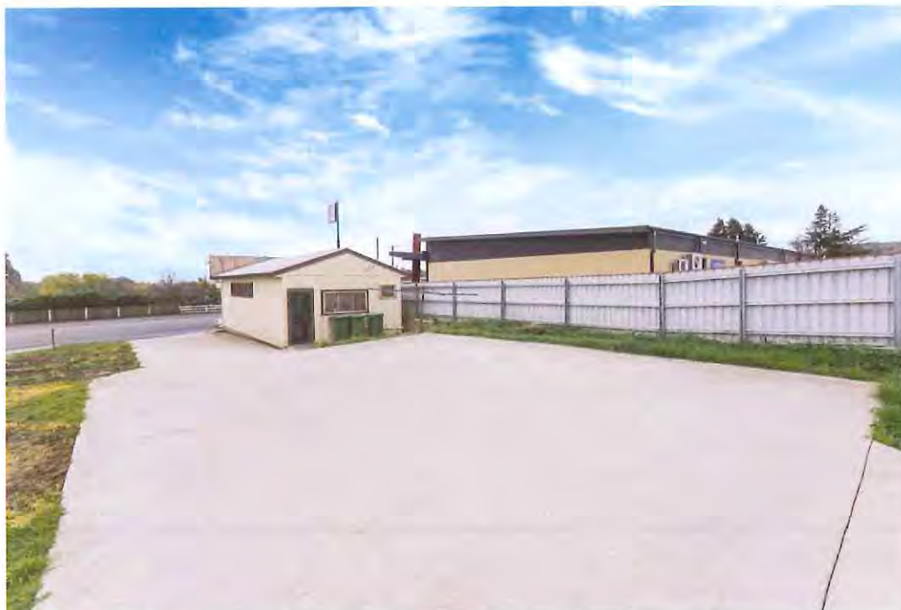
Figure 2: View of the Driveway and Hard Stand – from the East (Rear)
