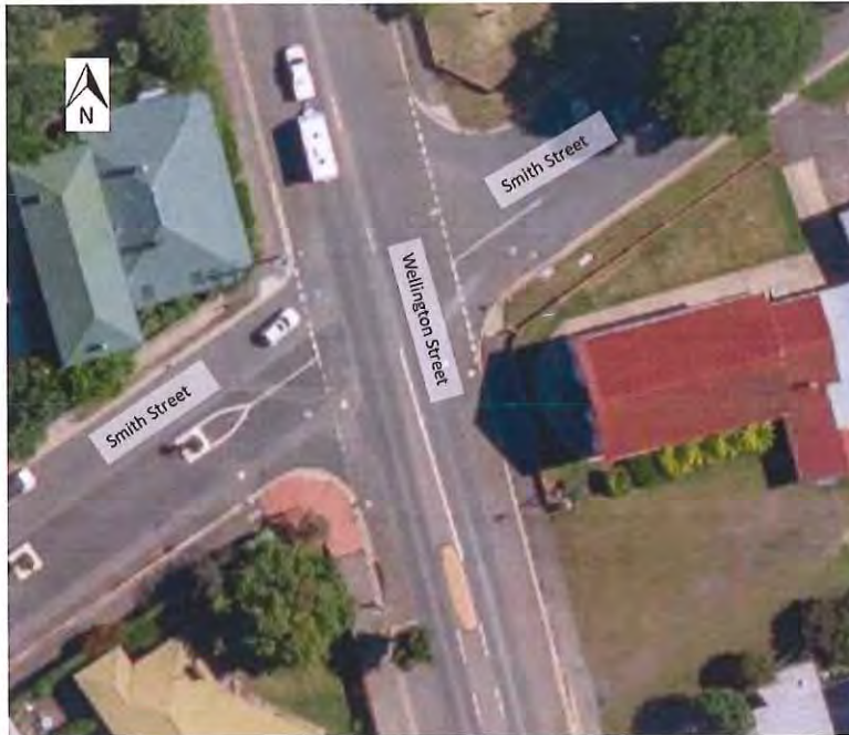
Figure 4: Wellington Street / Smith Street intersection (Aerial Source: theLIST)
