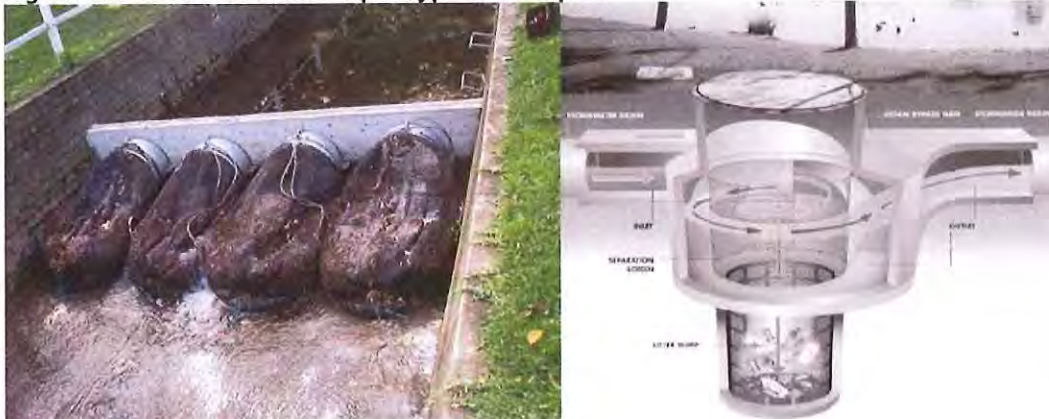
Figure 16: Gross Pollutant Trap – Typical Examples
