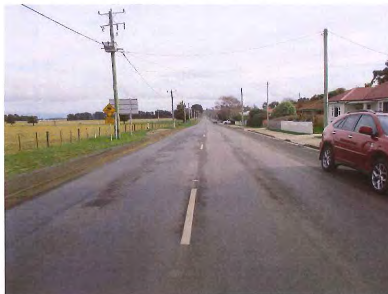
Photograph 4.2: View to west along Drummond Street
