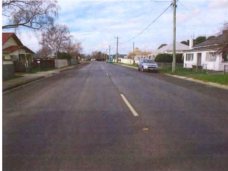
Photograph 4.1: View to east along Drummond Street towards junction with Main Road
