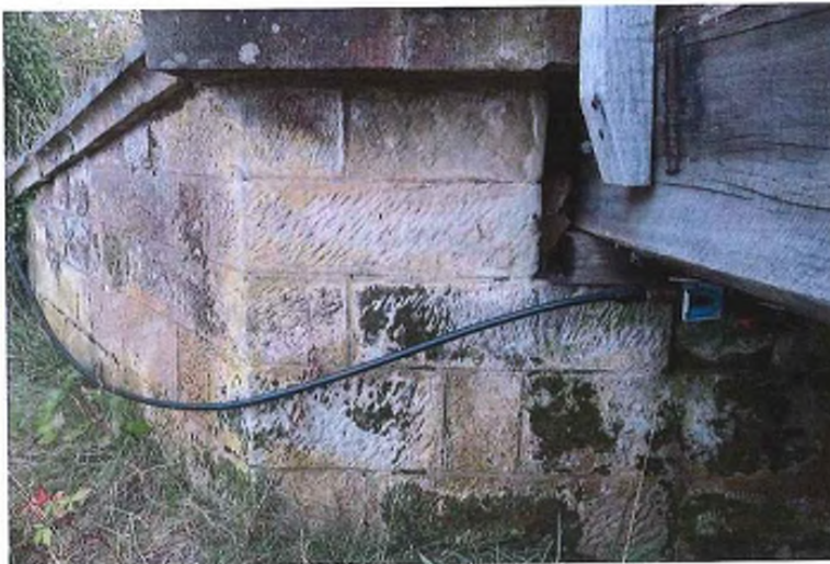
Figure 9: Face of northern abutment
