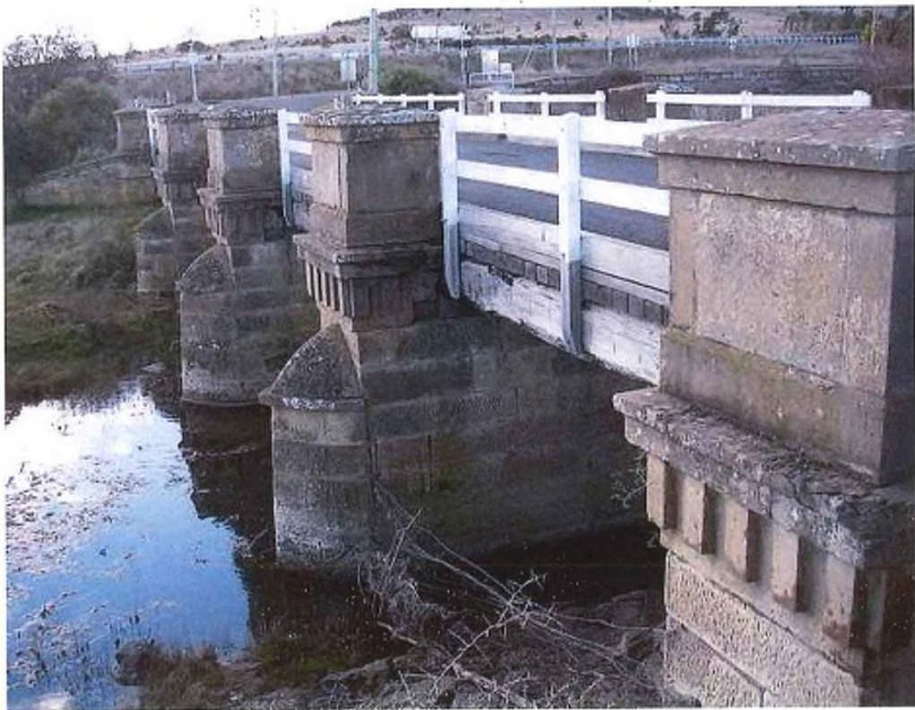
Photograph 2. View of detail of upstream face.
