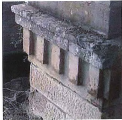
View of full width header stone in pier.
