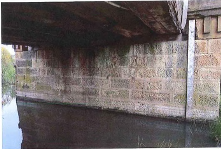
Figure 8: Southern face of the southern pier 1
