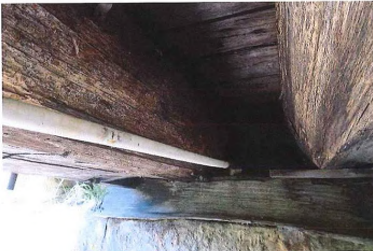
Figure 6: Timber girders and spreader at southern abutment
