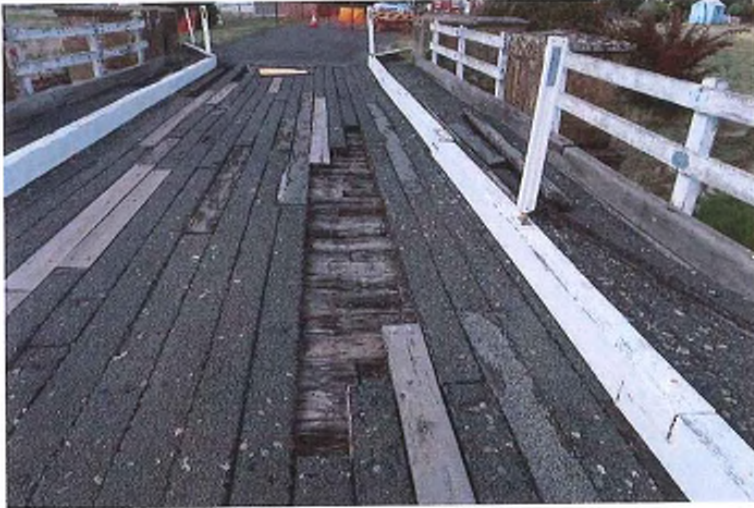
Figure 7: Deck condition
