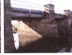
Timber deck and stone pier
