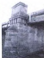
Tunbridge Bridge pier
