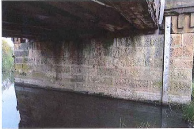
Figure 8: Southern face of the southern pier 1
