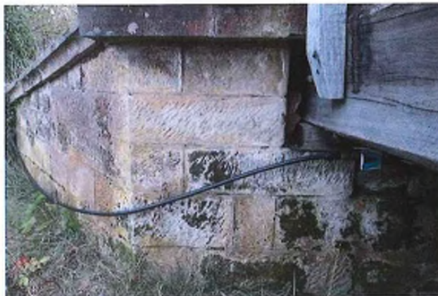
Figure 9: Face of northern abutment
