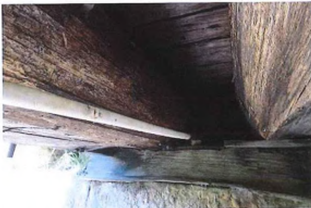
Figure 6: Timber girders and spreader at southern abutment
