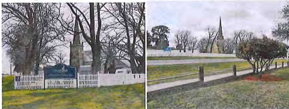
Figure 3: Existing Pale and private property signs
