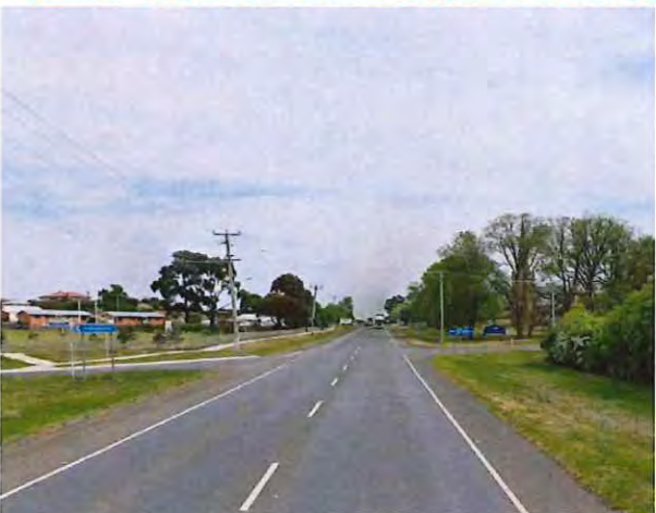
Figure 13 – High Street Southern approach to Bridge Street Intersection.
