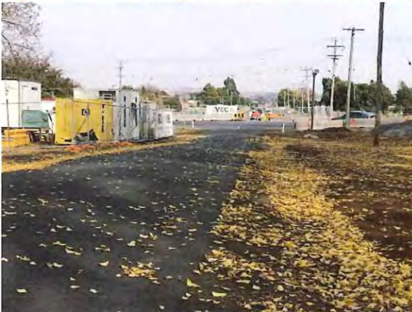
Figure 21 – Looking right along Bridge Street from proposed carpark
