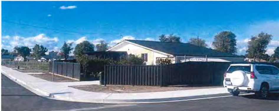
Figure 2 - existing colourbond fence.
