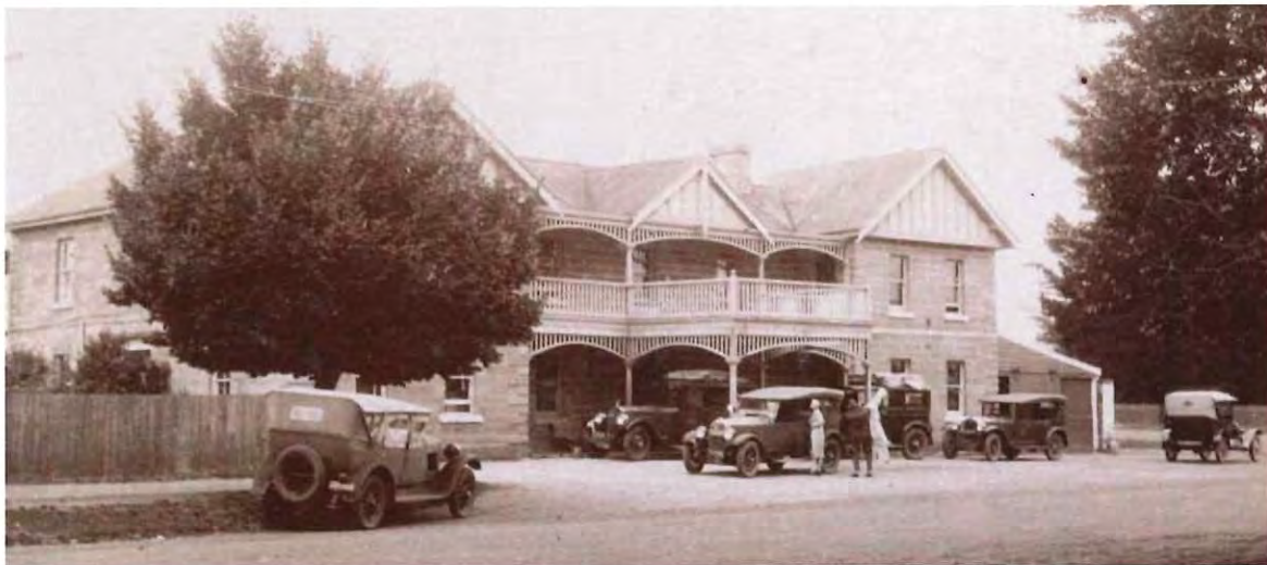
Figure 4.10 – 1932 photograph of the hotel. Harvey Collection, State Library of Victoria.
