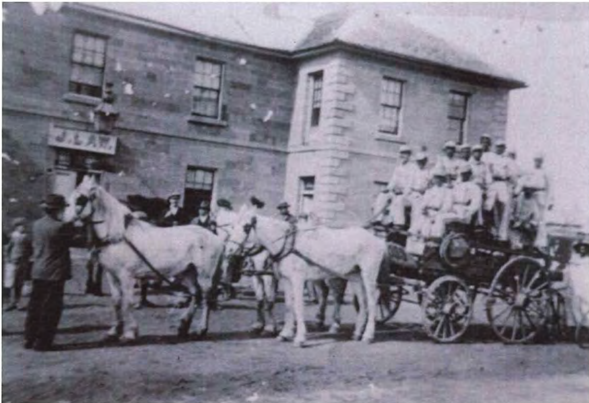
Figure 4.5 – A c1900 photograph of the hotel. Note the lack of veranda and balcony, and hipped roof form. Note also the door-sized window on the first floor – possibly anticipating a balcony from the outset?
