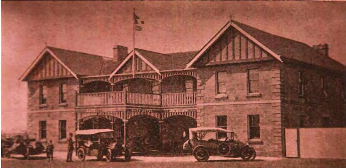
Figure 4.7 – A c1915 photograph of the hotel – under the ownership of Mr. Law the veranda, balcony and port-cochere were built and the hipped roof forms extended to forward facing gables with roughcast infill. Weekly Courier.
