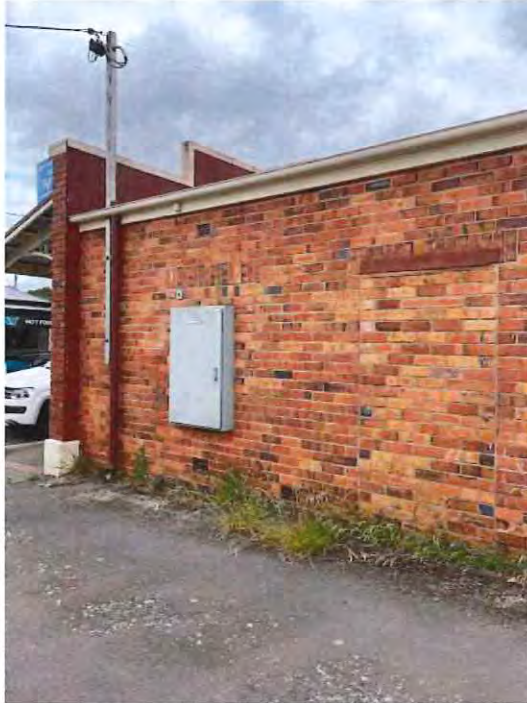
Fig.1 - Showing existing masonry wall and brick lintels.
