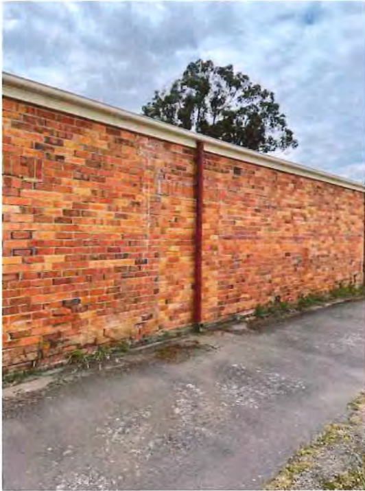
Fig.3 - Showing existing masonry wall and brick lintels.
