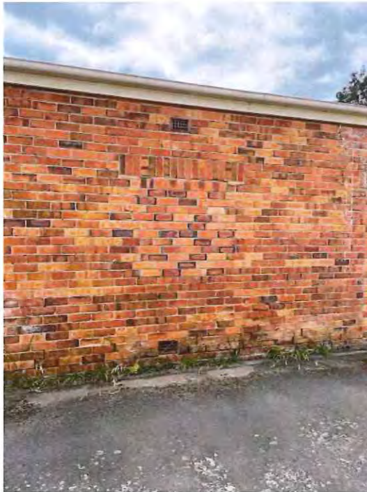
Fig.2 - Showing existing masonry wall and brick lintels.
