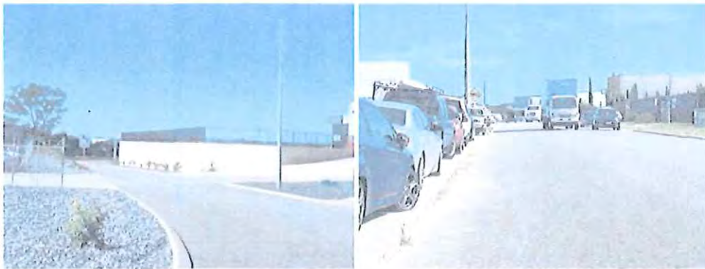
Figure 5 Bibra Lakes Industrial area - no footpaths
