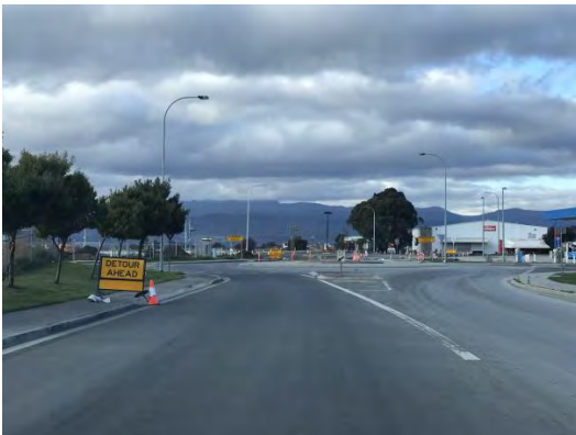
Figure 16 – Translink Avenue Western approach to John Street roundabout
