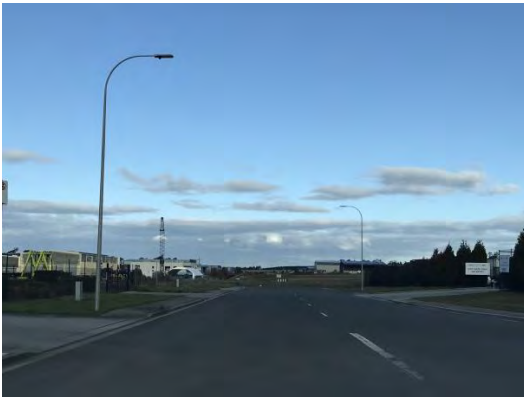
Figure 14 – Translink Avenue Northern approach to development site
