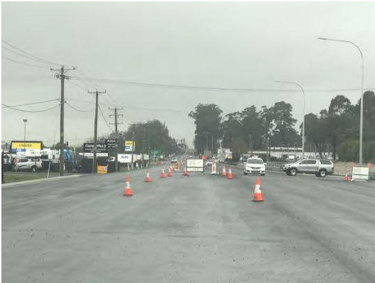
Figure 23– Evandale Main Road Northern approach at Boral Road
