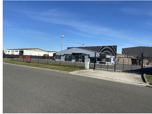
Figure 9 Subject site - north east elevation
