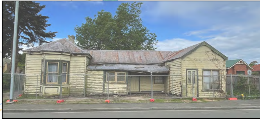
street elevation, photo taken Nov 2022
