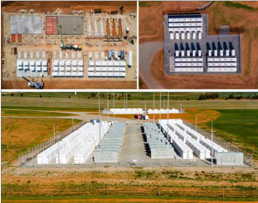
Figure 2: Hornsdale Power Reserve
