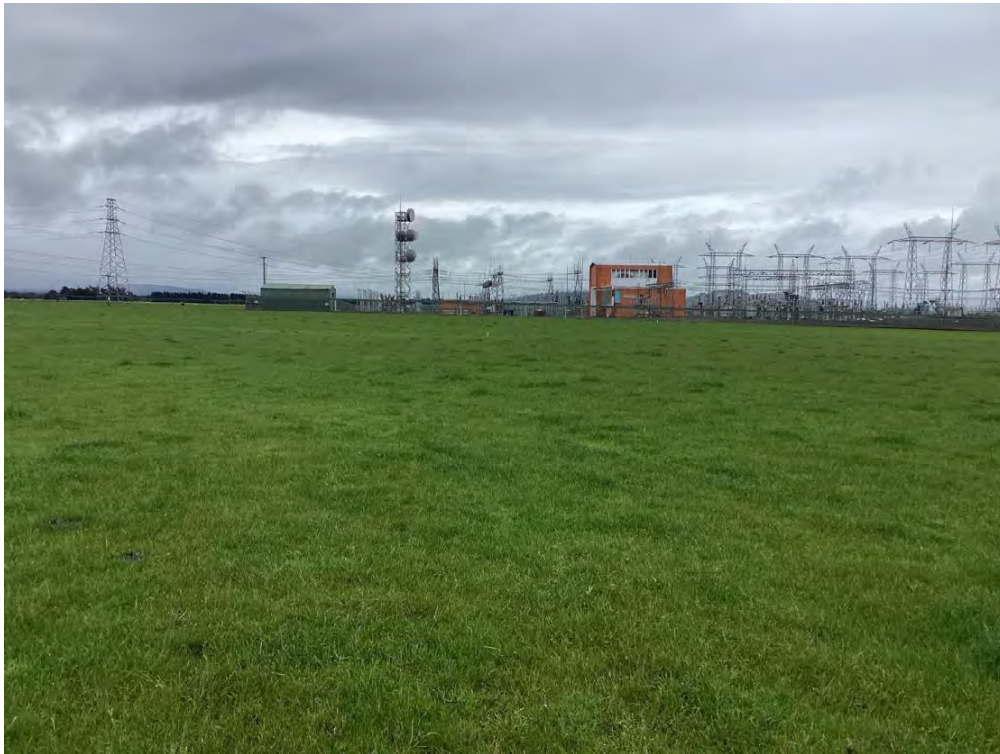
Figure A2-5: View east from Pit 3 south towards TasNetworks substation.
