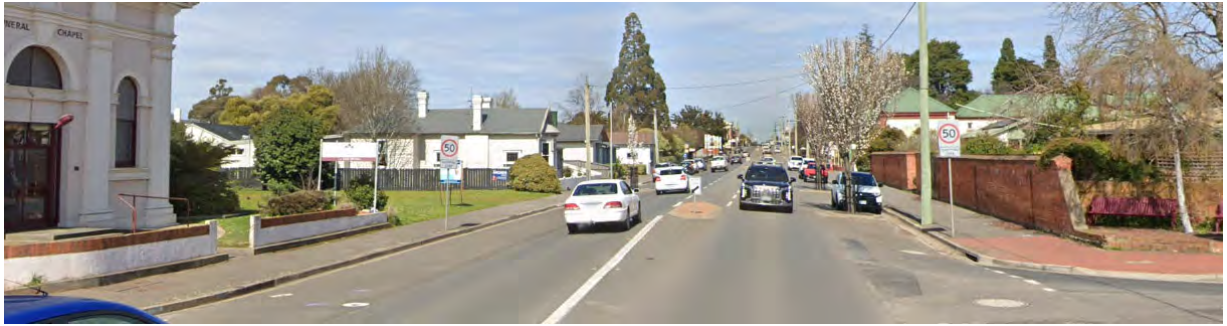
Figure 7 Wellington Street (looking south, Longford)
