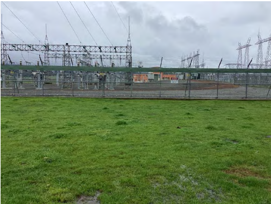
Figure A2-2: View west from Pit 1 towards TasNetworks substation.
