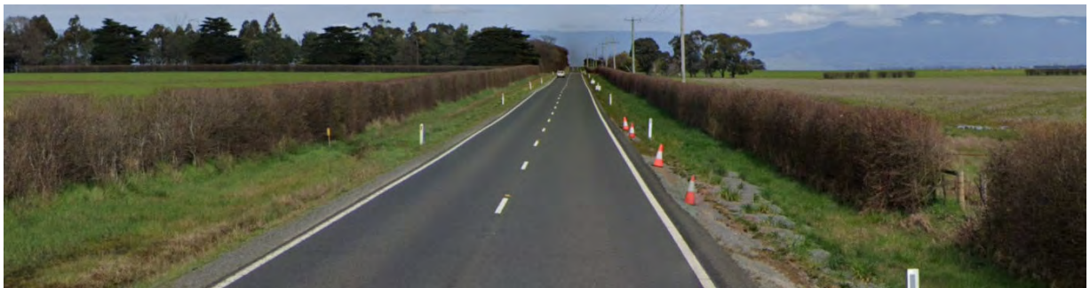
Figure 9 Cressy Road (looking south, Cressy)
