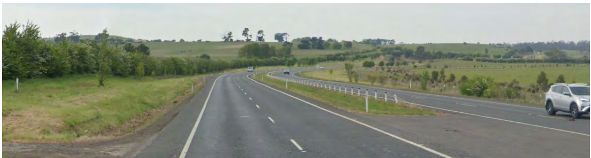
Figure 5 Midland Highway (looking southeast near Prospect)
