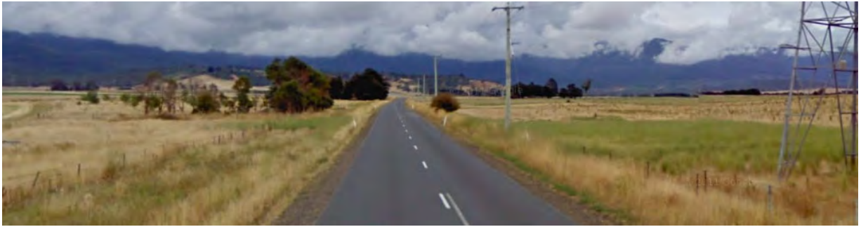
Figure 11 Poatina Road (looking west near the site access)
