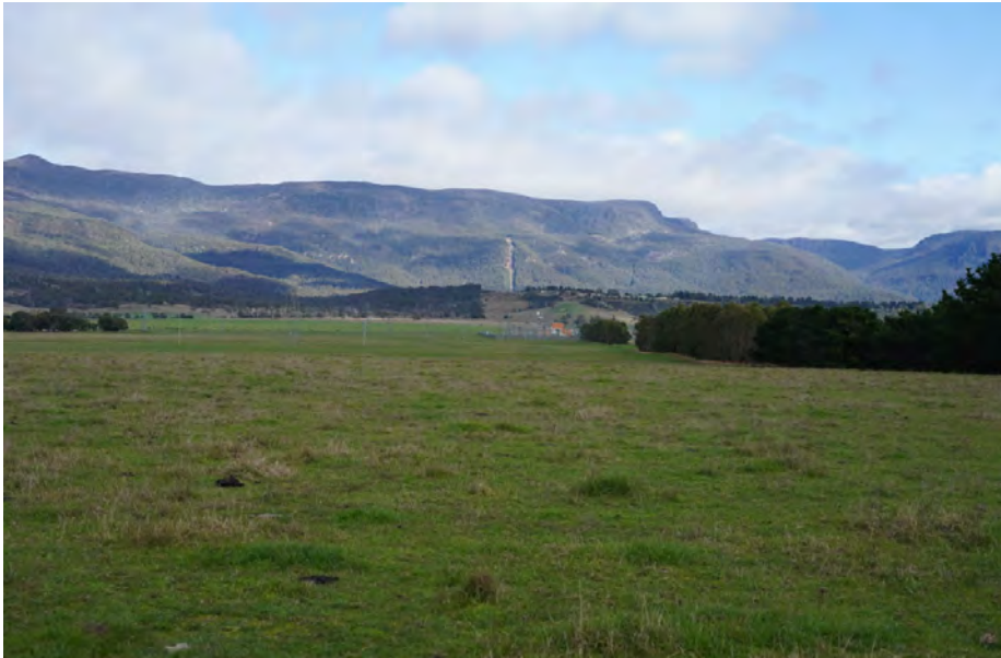
Photograph 4.1 View from Poatina Road west to Western Tiers and penstocks with the red brick of the two-storey building within the substation site visible (Source: Inspiring Place)
