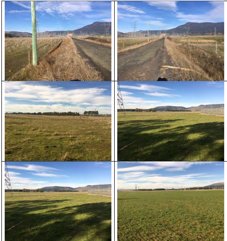
Figure 3. Top-The substation access road. Middle-Access across paddocks north and east of the substation. Bottom-The construction area for the battery project.
