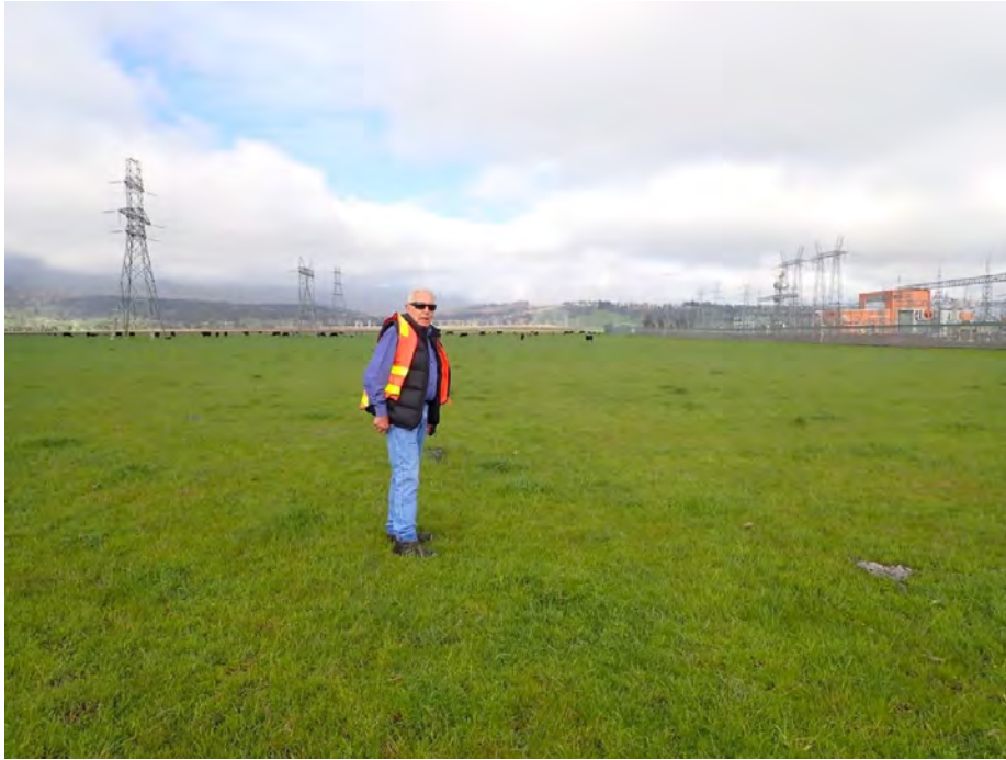
Plate 4: View west showing the Palmerston TasNetworks Substation (right) and pastureland within the study area.
