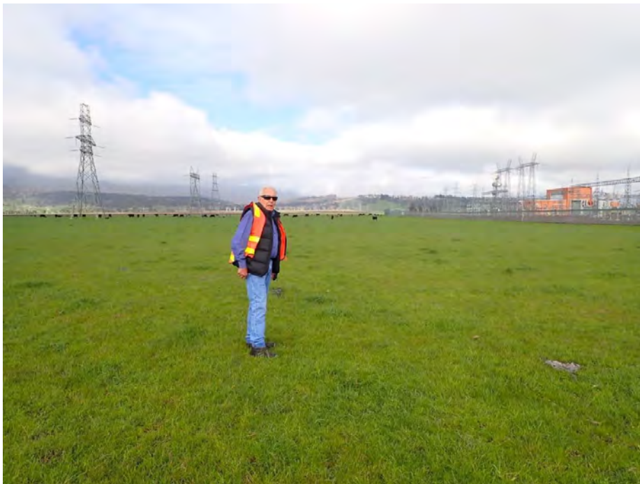
Plate 4: View west showing the Palmerston TasNetworks Substation (right) and pastureland within the study area.
