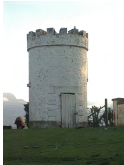
Castellated Tower at Woodside DPIPWE 2008
