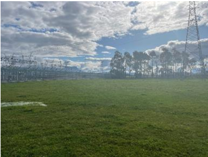
Photo 6: The approximate location of a section of the Right of Way, on the north-eastern side of the Palmerston Substation.
