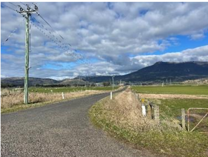
Photo 1: TasNetworks internal road viewed from the Poatina Road looking towards the Palmerston Substation.
