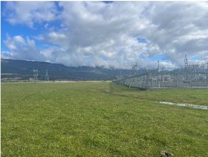
Photo 5: The approximate location of a section of the Right of Way, south of the Palmerston Substation.
