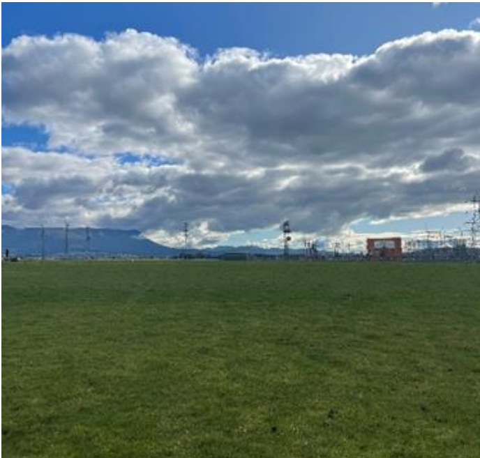
Photo 3: TasNetworks Palmerston Substation and battery storage location looking north west from the site.
