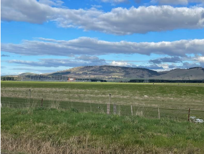
Photo 6: The view of the battery storage location from Poatina Road, looking in a south-easterly direction.
