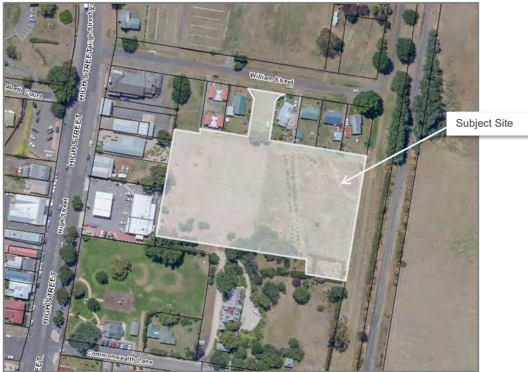
Figure 1 Aerial view of the subject site (Source: LISTMap)
