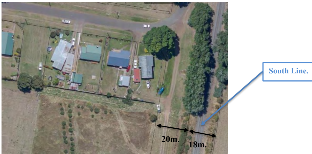
Figure 6 – South Rail Line adjacent the development site.
