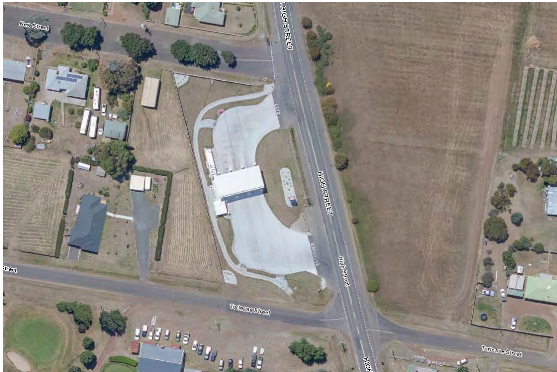
Figure 2 Campbell Town Truck Refuelling Station
