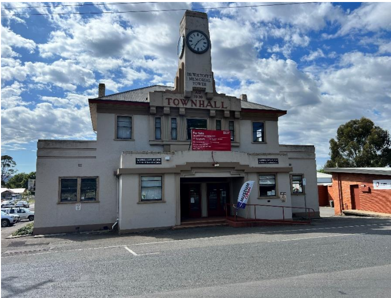
Photograph 1: View of the front of the Campbell Town Hall from High Street
