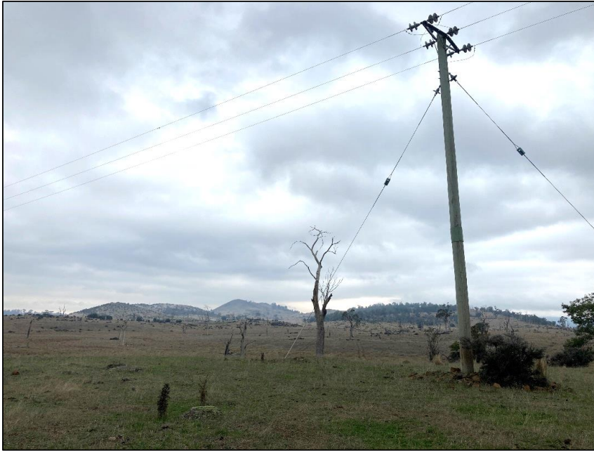
Image 9. Overhead powerlines and electric pole near proposed development site (taken at site assessment on 29/04/22).
