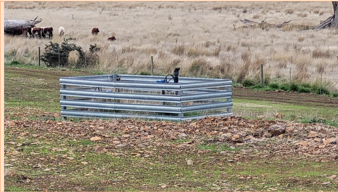
Location of proposed water connection point from existing static supply of dam
