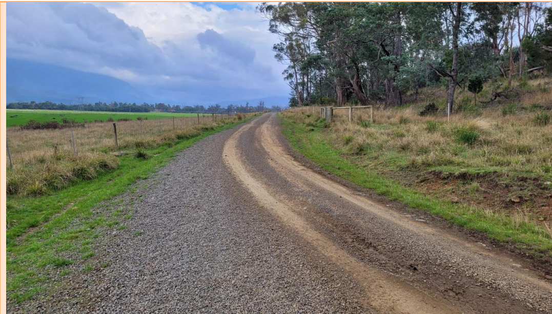
Existing access (3.5m wide approx.)
