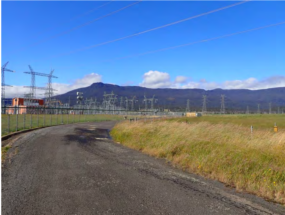
Plate 5: View southwest showing the graded access track in the study area.
