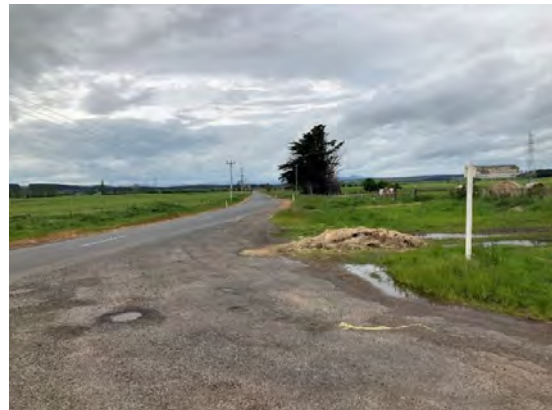
Figure 8: Poatina Rd, east approach to Palmerston Substation Access Rd
