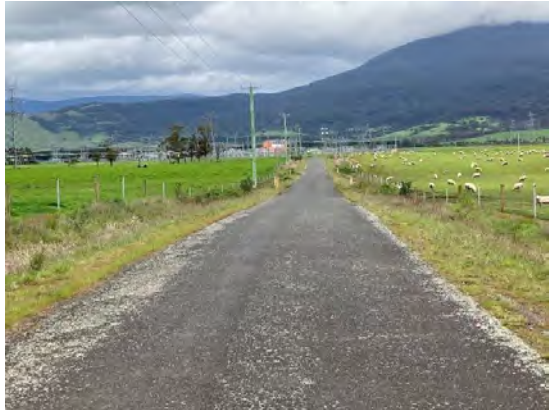
Figure 5: Palmerston Substation Access Road (looking south)
