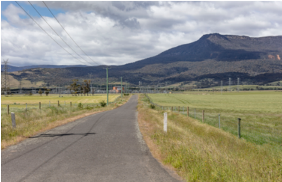
Figure 22 - KOP 2: Approx 4554 Poatina Rd, corner of unnamed road, entrance to substation, facing approx 170 Degrees South to target. Taken at 11:17am EST on 28/11/2022. Canon EOS 5DSR, 50.6 MGPXL Full Frame Digital Camera at 50mm Focal length.
