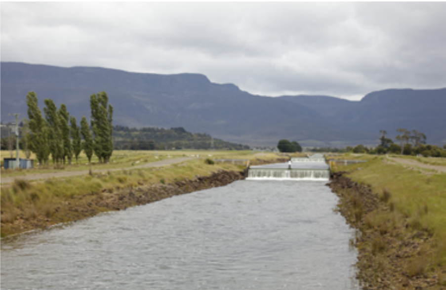
Figure 27 - Photograph of Tail Race. Taken at 11:11am EST on 28/11/2022. Canon EOS 5DSR, 50.6 MGPXL Full Frame Digital Camera at 65mm Focal length.
