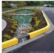
Rain gardens to kerb buildouts.
