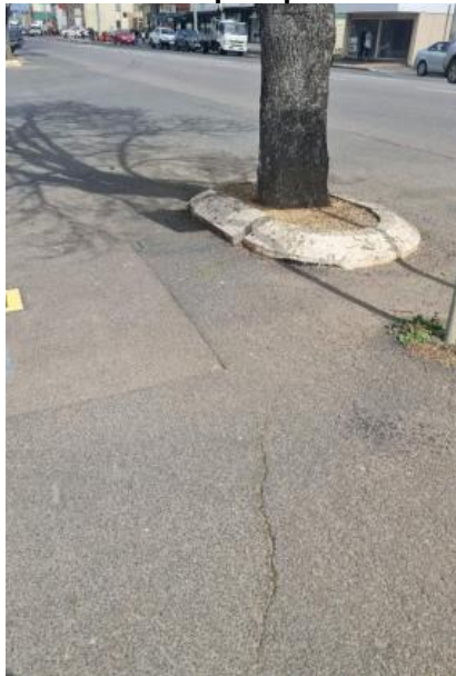
Photo 10 – Car park pavement
