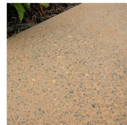
Exposed coloured concrete pavement.
