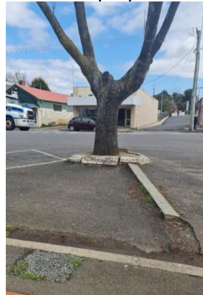
Photo 12 - Car park pavement
