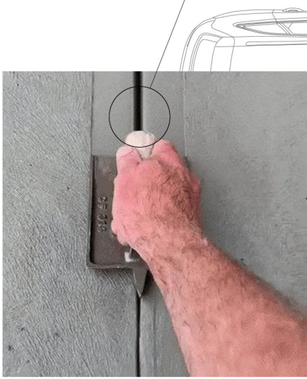
Troweled joint patterning.
