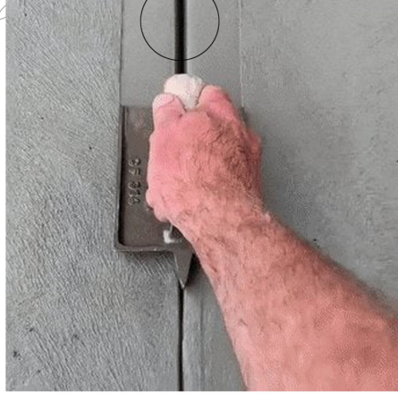
Troweled joint patterning.
