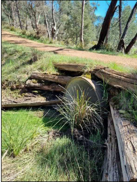
Figure 2: DN1200 RCP Culvert
