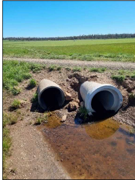
Figure 3: Twin DN600 RCP Culvert
