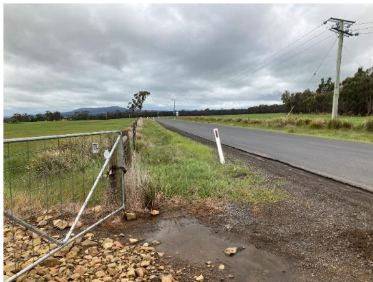
Figure 12: Macquarie Rd, west approach to Access #1
