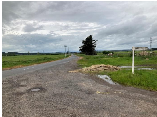
Figure 45: Poatina Rd, east approach to Palmerston Substation Access Rd
