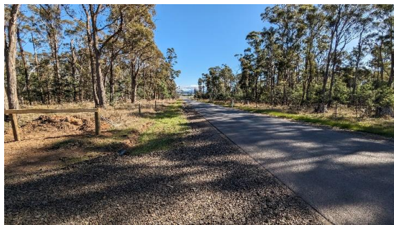
Figure 21: Macquarie Rd, west approach to Access #4
