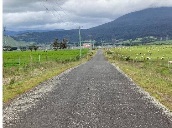
Figure 43: Palmerston Substation Access Road (looking south)
