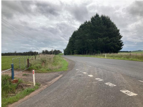
Figure 27: Macquarie Rd, west approach to Lake River Road
