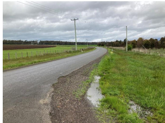
Figure 25: Macquarie Rd, east approach to Connorville Rd
