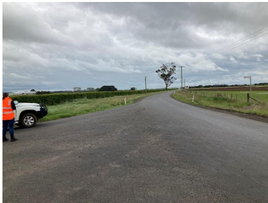
Figure 24: Macquarie Rd, west approach to Connorville Rd
