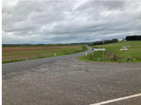
Figure 28: Macquarie Rd, east approach to Lake River Road
