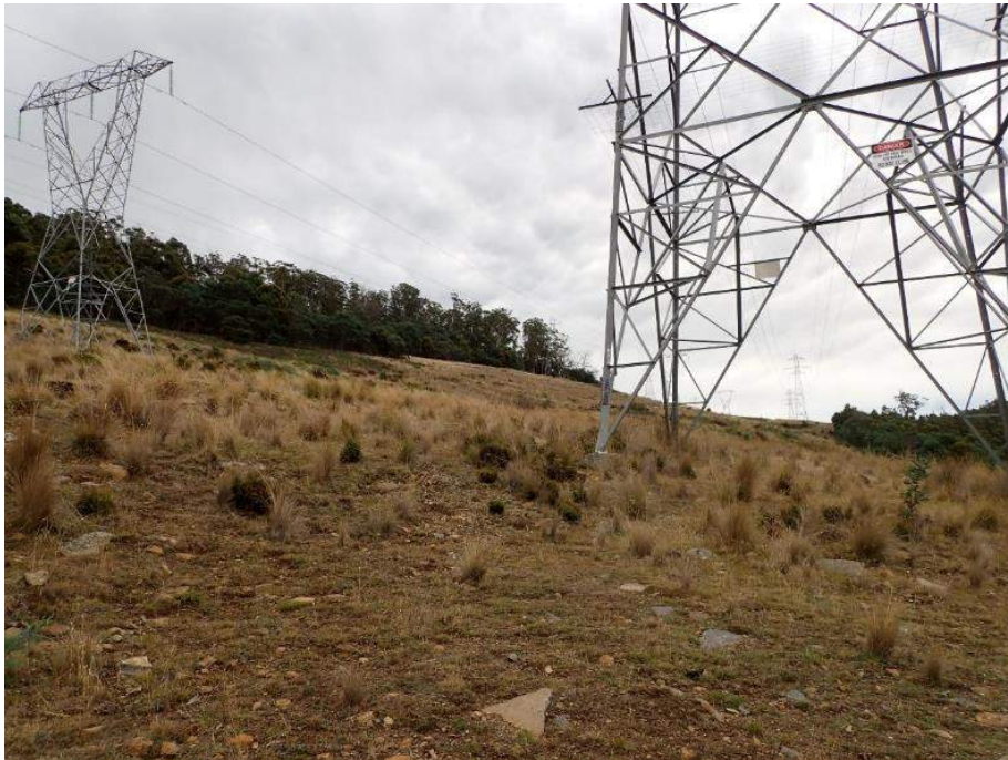
Plate 6: View northwest showing 40° slopes and existing transmission line within the study area.
