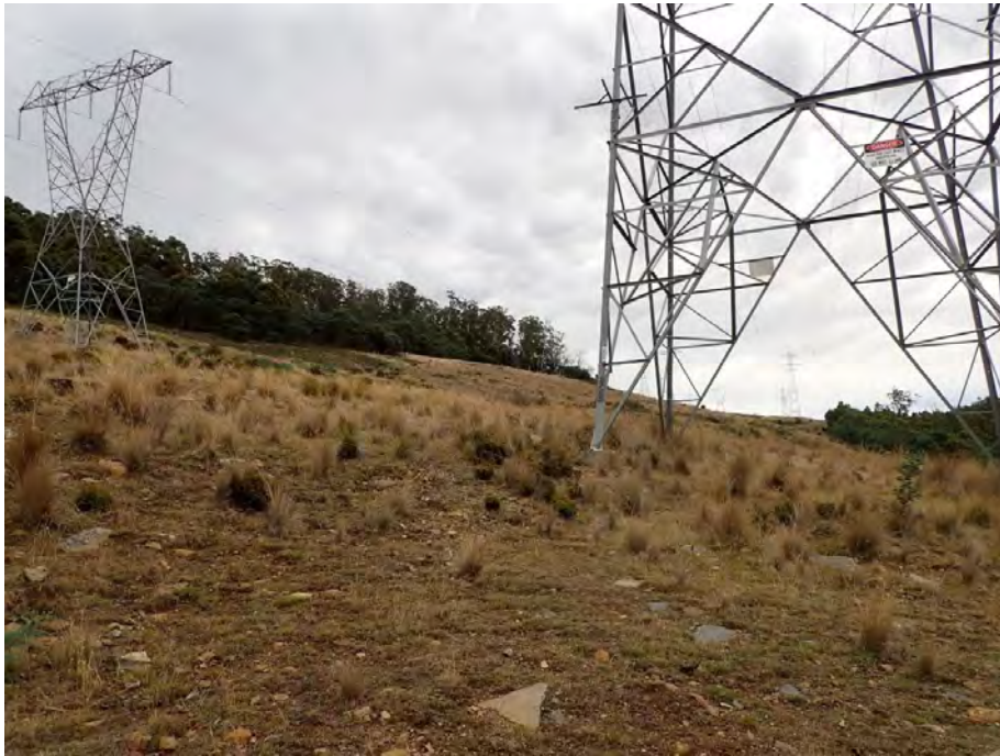
Plate 6: View northwest showing 40° slopes and existing transmission line within the study area.
