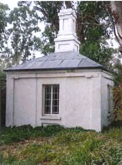
Gate house, Clairville DPIPWE 2014
