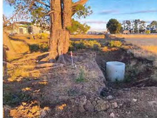
Figure 3. Image showing open trench inside the trees SRZ.
