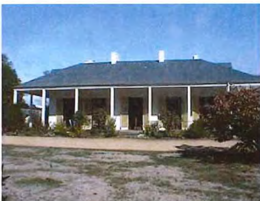
Verandah, Clairville DPIPWE c2002
