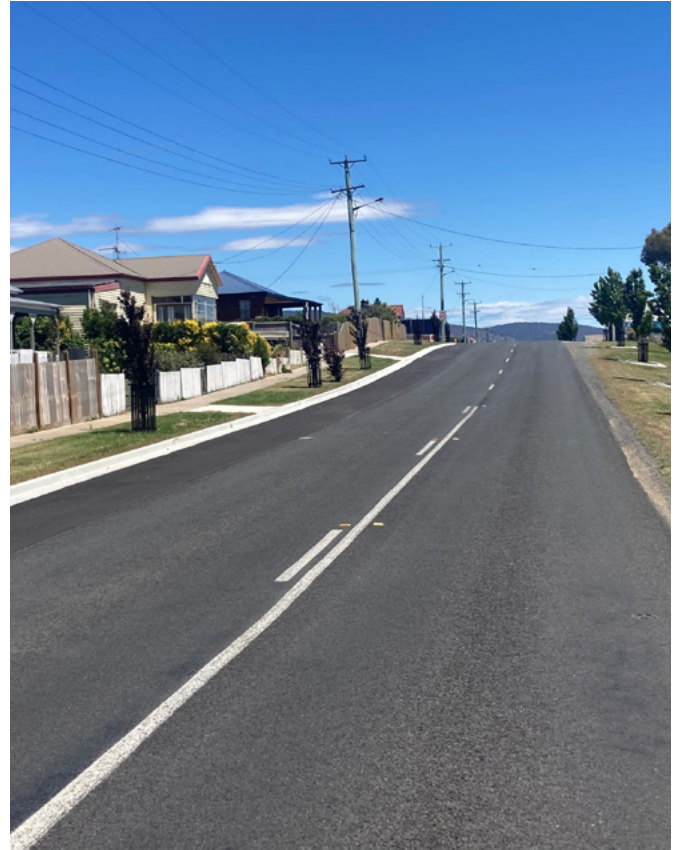
• Kerb and channel construction Falmouth Street, Avoca
