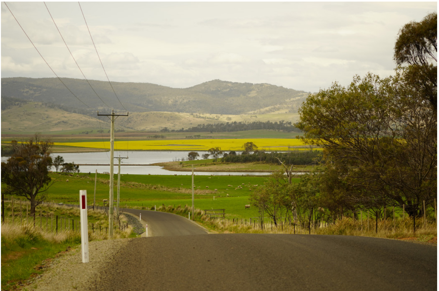
• Glen Esk Road construction
