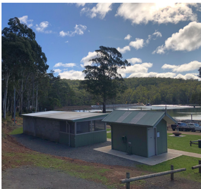
• Lake Leake Amenities
