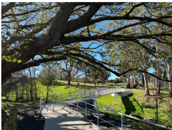
• Footbridge at Perth's William Street Reserve
