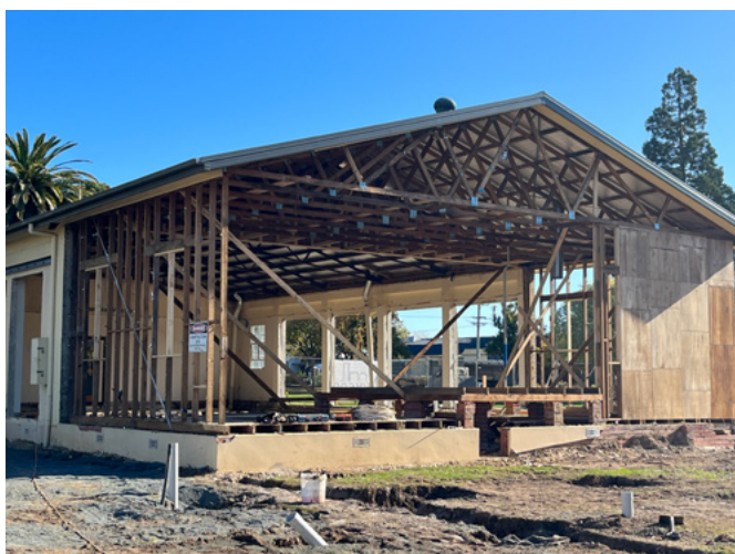
• Upgrade of Longford's Memorial Hall under construction
