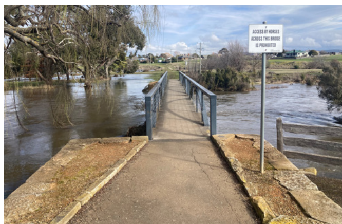
• Flooding at Bridge Street, Campbell Town
